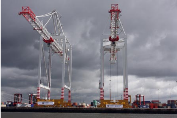
New gantry cranes at DP World Southampton
