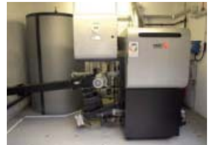
Woodfuel boiler at QECF
